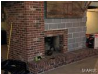
Wood burning located in basement
