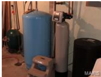
Back flush water filter, pressure tank, water softner
